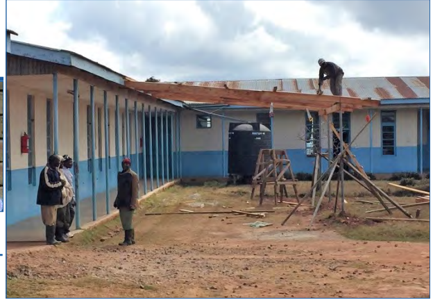
The roof of a new car-port being built at Milo hospital, Tanzania
